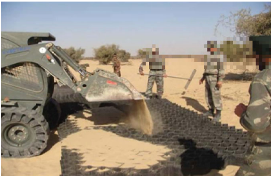
Fig. 12.14 Mechanical and manual filling of geocells with sand
