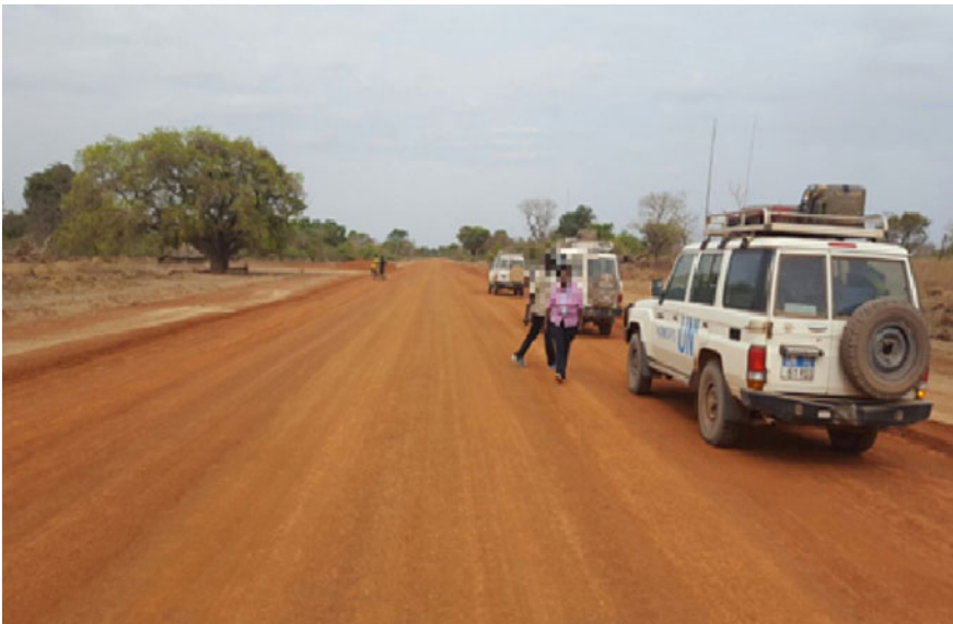
Fig. 15.8 Neoloy Geocell-reinforced rural feeder road, UN. Photo Credit UNOPS
