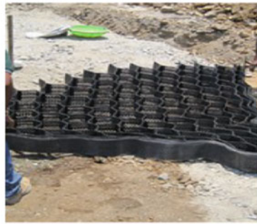
b Instrumentation and construction of reinforced section
