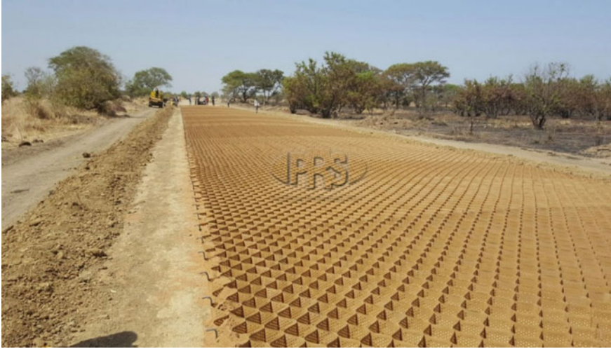
Fig. 15.7 Installation of Neoloy Geocell on rural feeder road project, UN. Photo Credit UNOPS
