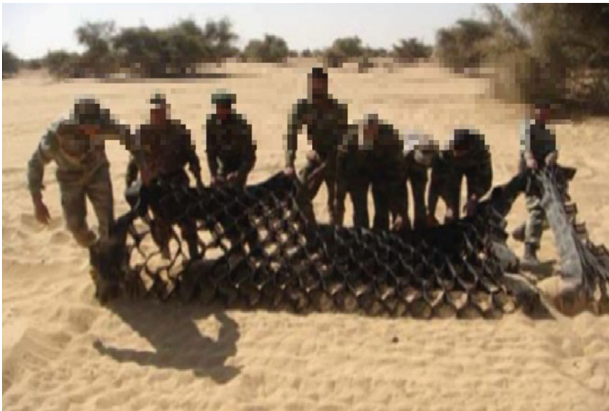
Fig. 12.18 Recovery of geocells using manual means
