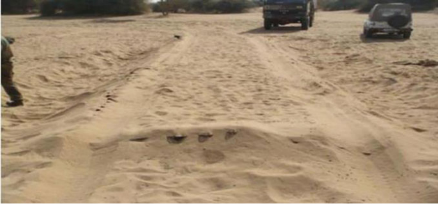
Fig. 12.15 Finished track with sand cover
