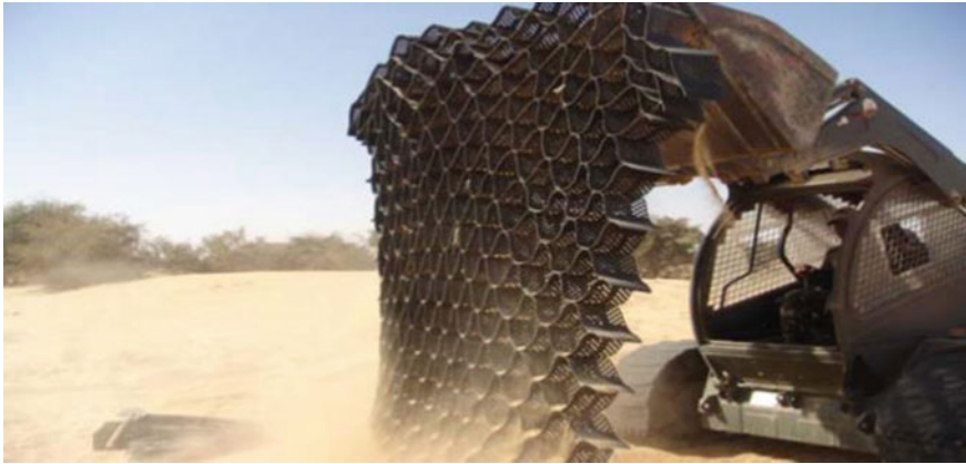
Fig. 12.17 Recovery of geocell using mechanical means
