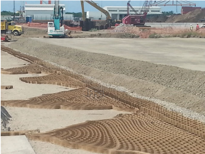
Fig. 15.19 Installation of Neoloy Geocells on subgrade of LTP. Photo credit Innovator
