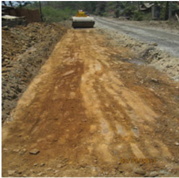
a Excavation of existing pavement, preparation of site with instrumentation (TPCs)
