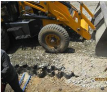
c Construction of geocell reinforced GSB layer and load test
