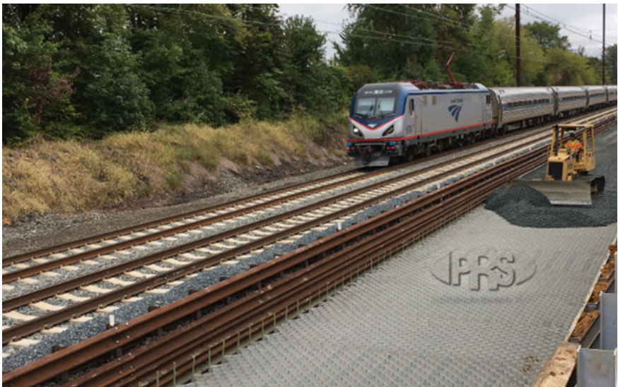
Fig. 15.13 Installation of Neoloy Geocell stabilized track (rebuild). Photo Credit PRS Geo-Technologies
