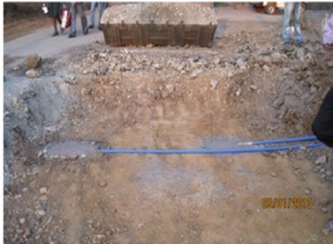
a Excavation of existing pavement, preparation of site with instrumentation (TPCs)
