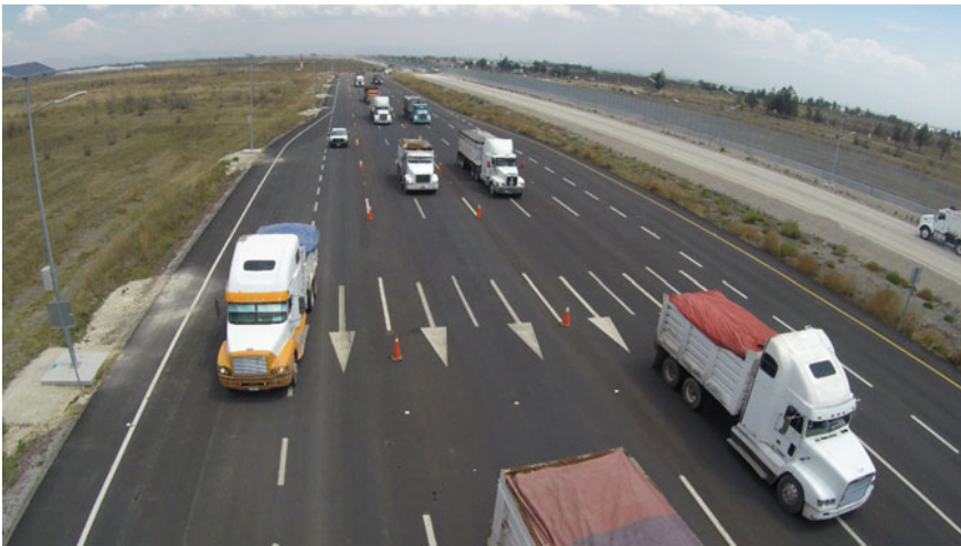
Fig. 15.2 Neoloy Geocell stabilized asphalt pavement roadways. Photo credit Innovater
