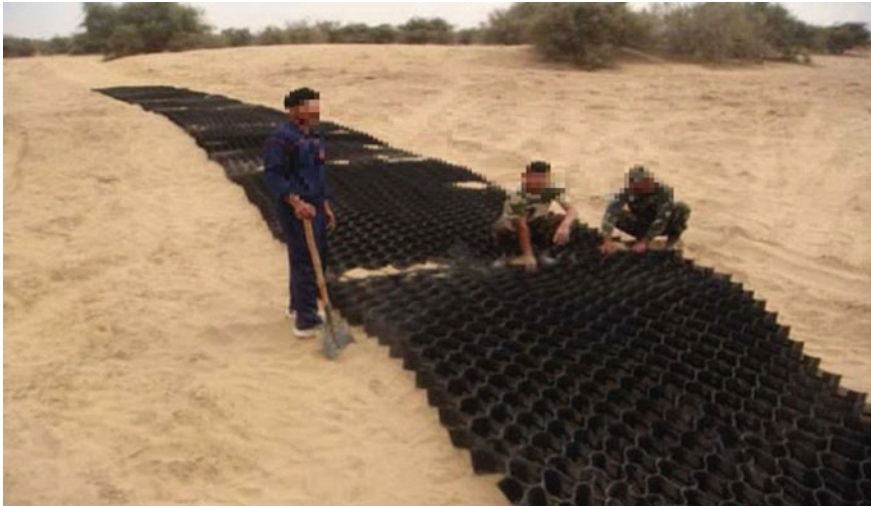
Fig. 12.13 Laying of geocell over 30 m stretch
