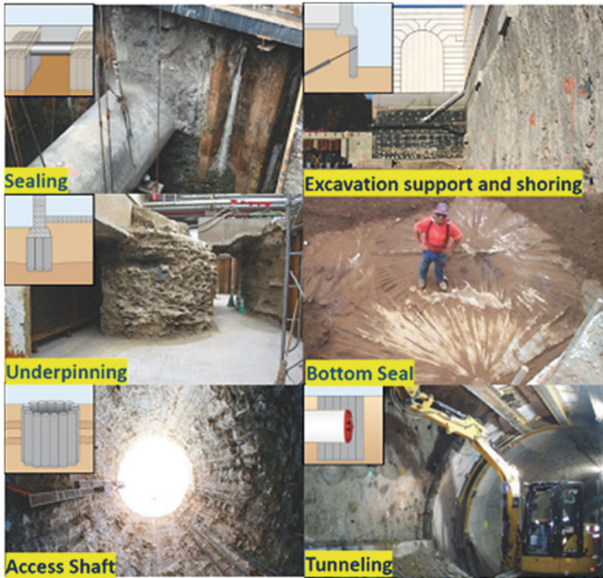
Fig. 2 Applications of jet grouting ( credited to Hayward Baker Inc.)
