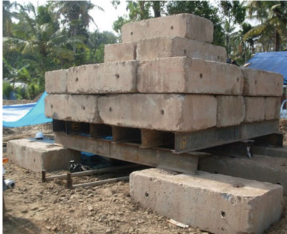
Fig. 10 Typical “reaction kentledge” for load test over stone column
