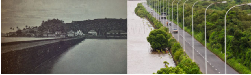
Fig. 5 Ribandar causeway in 1950 and 2001, Goa
