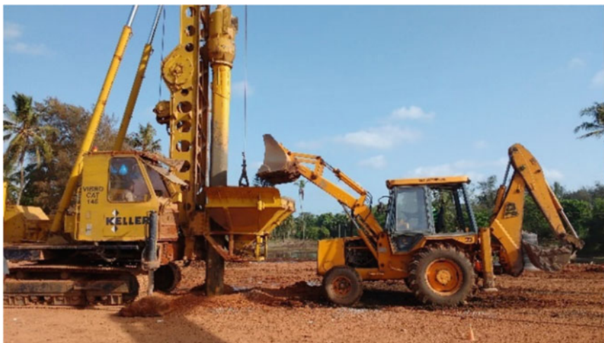
Fig. 5 Installation of vibro stone columns (dry bottom feed method)
