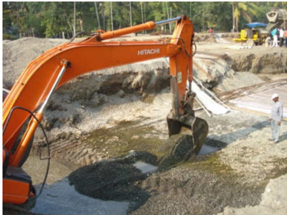
Fig. 7 Typical laying process of granular blanket
