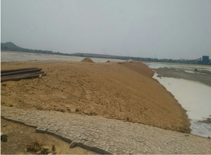
Fig. 16 Construction of first stage raising of ash bund
