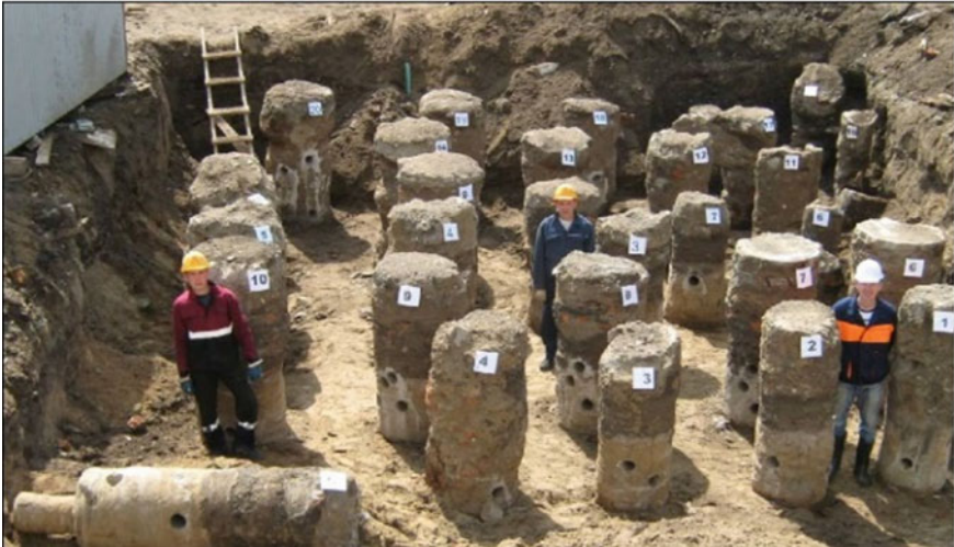
Fig. 5 Installed trial columns
