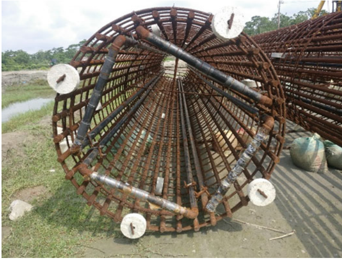
Fig. 11 Site photo showing reinforcement cage with grout pipes
