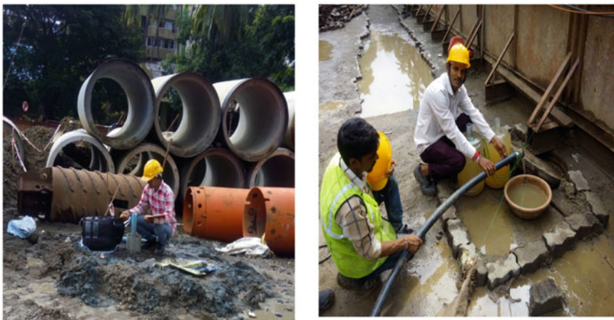
Fig. 11 Pump out test at Cuffe Parade station area
