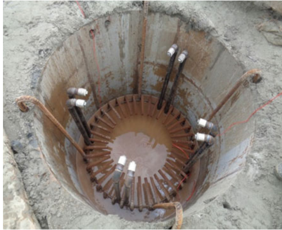
Fig. 9 Site photo showing grout pipes on test pile
