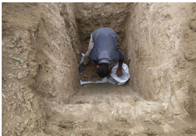
Fig. 2 Collection of representative sample from a borrow area pit
