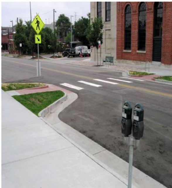
Fig. 5 Advanced sidewalks for pedestrians [4]
