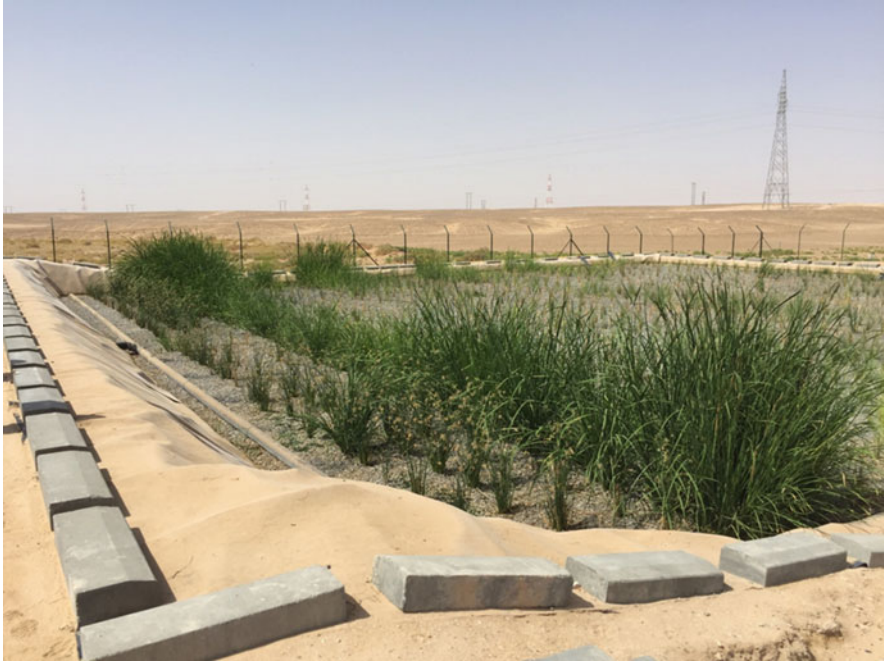
Fig. 7.4 The second-stage horizontal subsurface flow aerated constructed during the second month of operation. (Courtesy of Bauer Nimr LLC)
