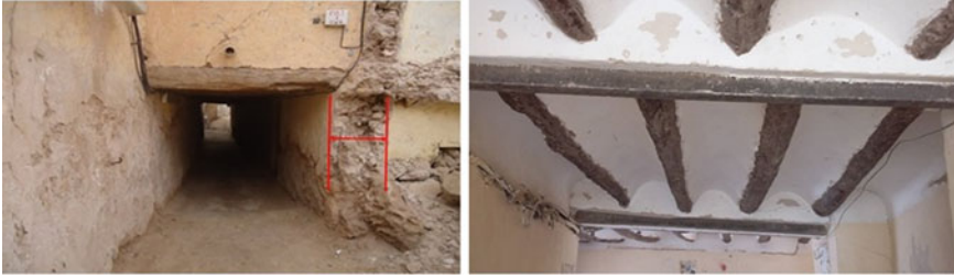
Fig. 74.6 Traditional massive roof and wall
