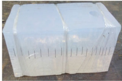
(f) Mould ready for casting
