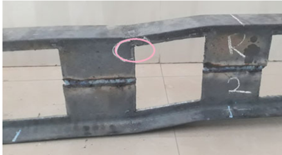
Fig. 6 A crack developed at the corner of rectangular web opening CSBIR 2
