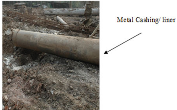
Fig. 11 Metallic steel Casing/Liner to prevent soil side collapse during pile construction
