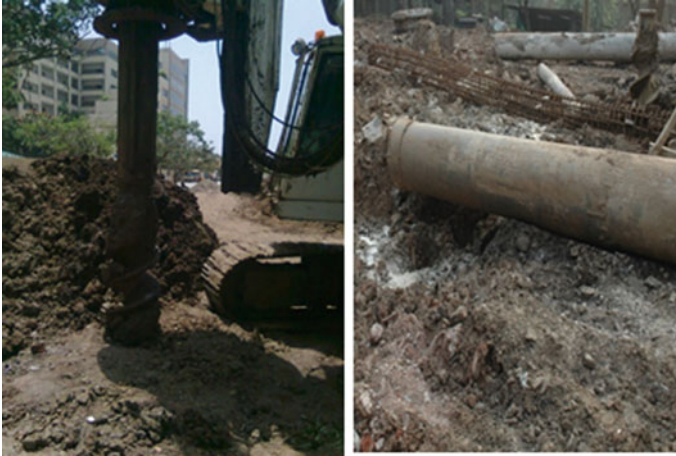
Fig. 4 Construction pile foundation by rotary drill methods
