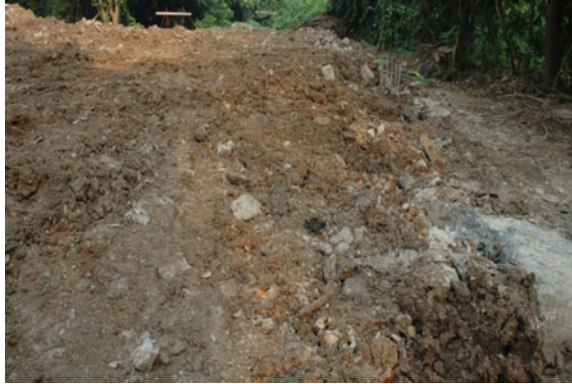
Fig. 7 Identification of pile locations during pile construction
