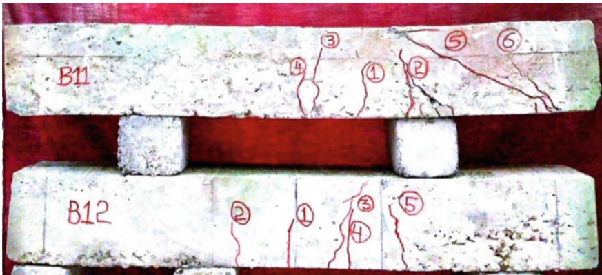
Fig. 11 Crack pattern for conventional beams
