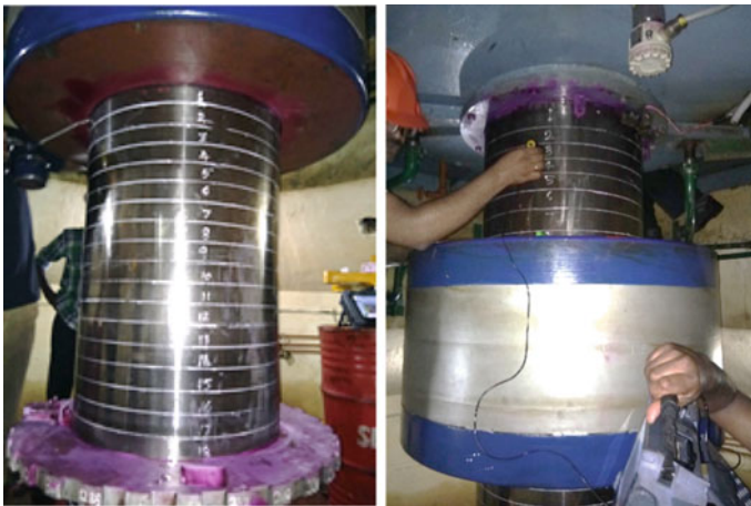
Fig. 4 Patching made on turbine and generator shaft region for paut
