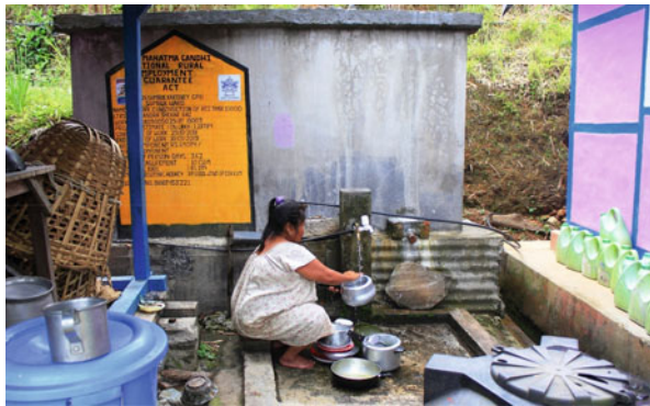
Fig. 2.9 Water storage tanks are a viable option for households located on the ridge top. Spring water and rooftop rainwater can be channelized into these reinforced concrete tanks having 10,000 litre capacity and built with an investment of USD 19,000 each
