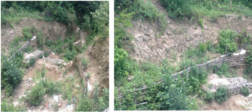
Fig. 3.5 Construction of bioengineering-based gabion wire check dams to control gully erosion
