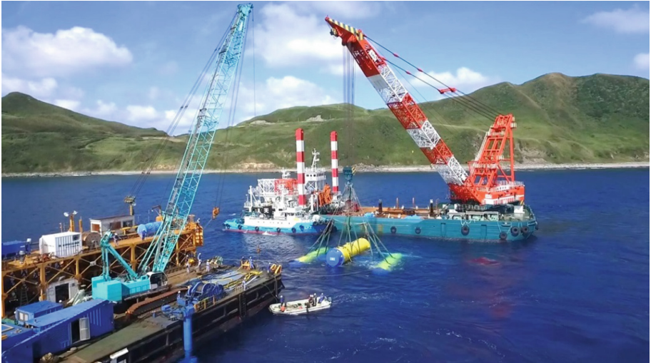
Fig. 17. Installation beside Kuchinoshima Island
