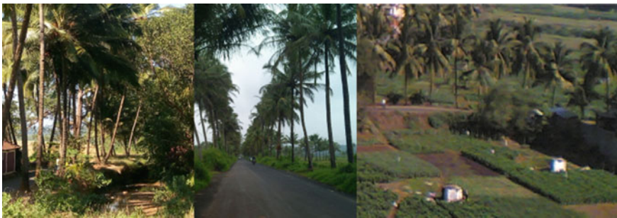
Fig. 1 Typical TGSB bunds used for transportation infrastructure in Goa
