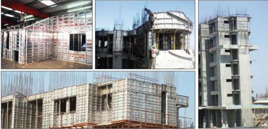
Fig. 1 Sample Mivan formwork
