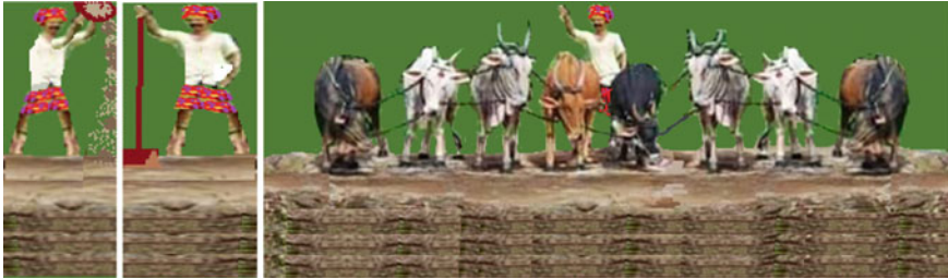
Fig. 5 Compaction of soil using traditional bullock chain and hand tamping
