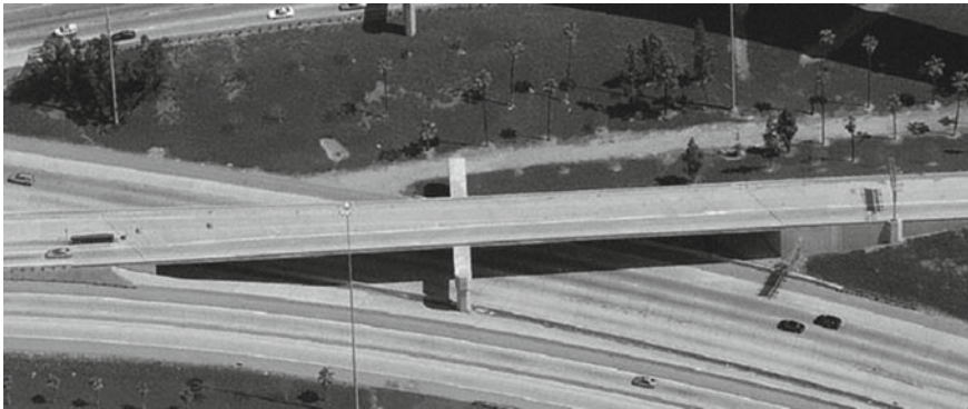
Fig. 7 91/5 Highway Overcrossing. Source Agrawal et al. [1]
