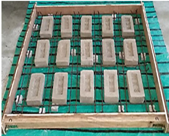
Fig. 3 Arrangement of RBC slab prior to casting
