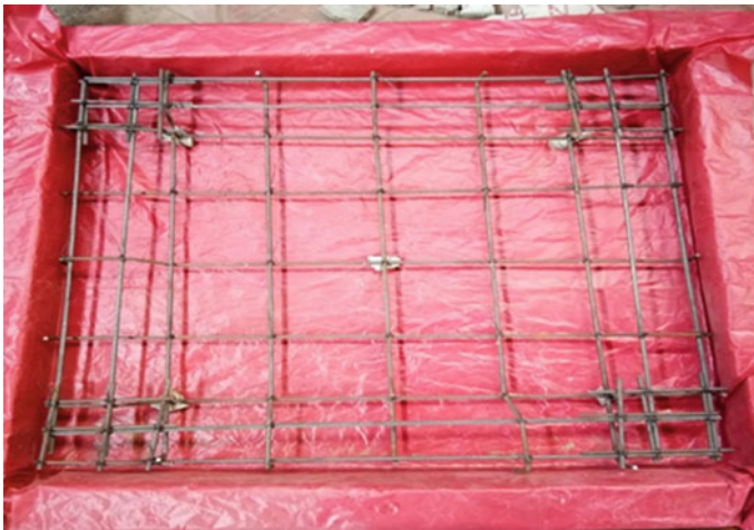
Fig. 1 Reinforcement cage for slab
