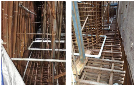
Fig. 2 Cooling pipes system of Part 1
