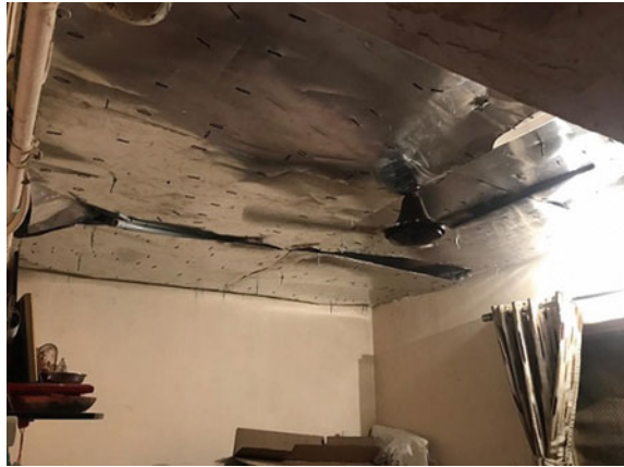
Fig. 12 Final assembly of panels
