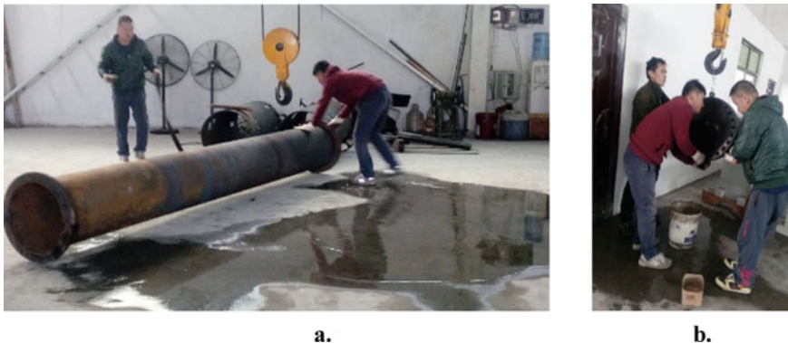
Fig. 1 a Hydrostatic test preparation on a 4 m length tube; b both ends of the tube are given a flange and closed with a round plate
