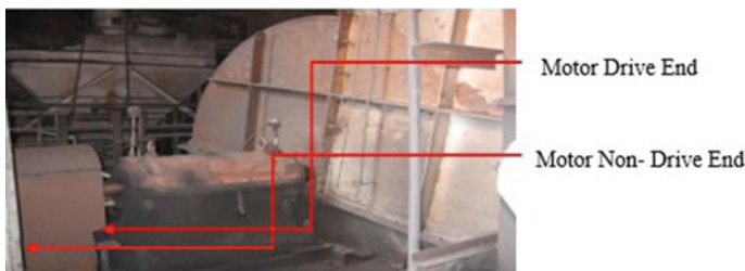
Fig. 1 Measuring points to collect vibration data from induction motor
