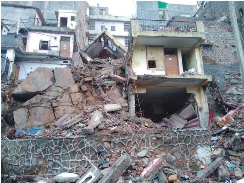
Fig. 16.2 Building collapse in Munirka Village on 23 February 2020 even in absence of tectonic activity underscores high vulnerability of physical infrastructure due to high rise building constructions on weak foundation. (Source: Author's)
