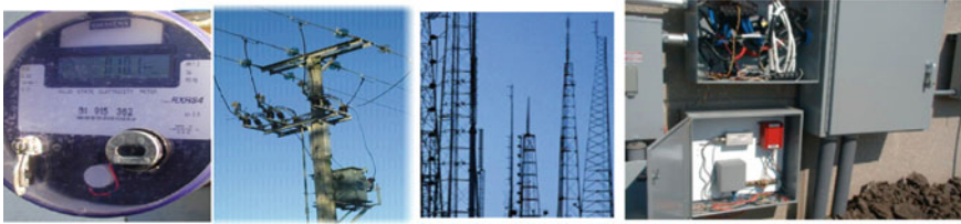
Fig. 7 Major facility of AMR/AMT company
