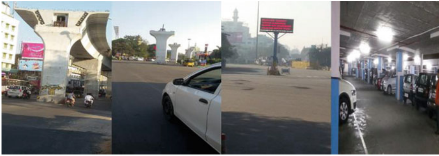
Fig. 1 Probable locations of vehicle and structural impact
