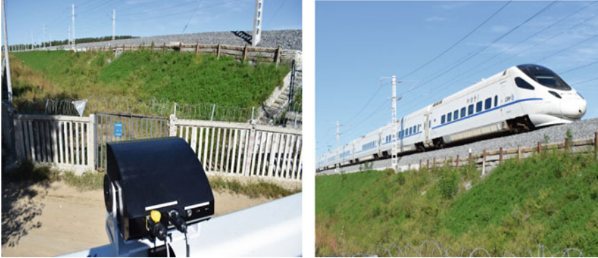
Fig. 2 Actual monitoring scene of the railway subgrade
