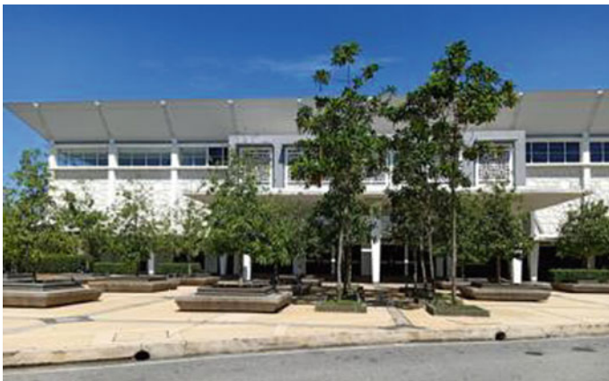
Fig. 22.4 Seating area outside the multipurpose hall
