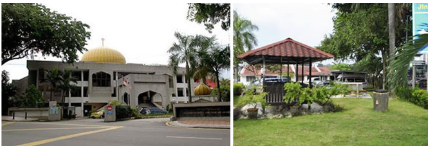
Fig. 22.12 The main entrance and recreational space of the mosque
