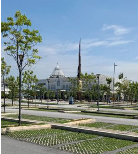
Fig. 22.3 View of car park provided for the congregation
