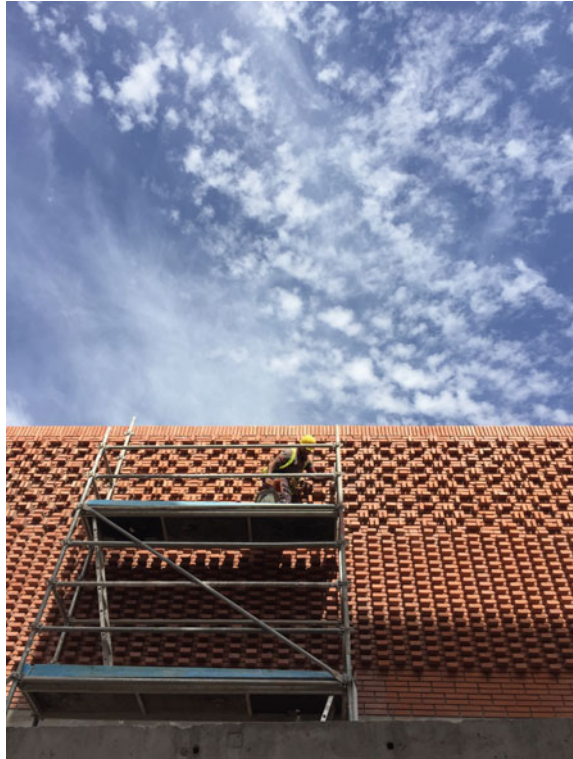
Fig. 6 YSL museum brickwork during construction. Photo courtesy: F. Tiaiba, 2017 ©
