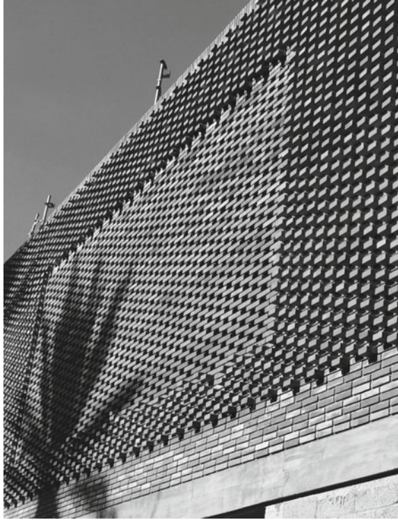
Fig. 16 Rear brick-pelt of the YSL museum. Photo courtesy: F. Tiaiba, 2017 ©
