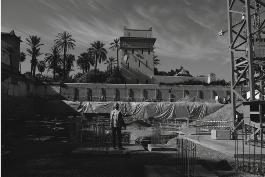
Fig. 7 YSL museum construction site. Photo courtesy: F. Tiaiba, 2017 ©
