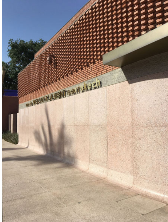
Fig. 3 YSL museum’s brick and terrazzo façade. Photo: A. Condello, 2019
