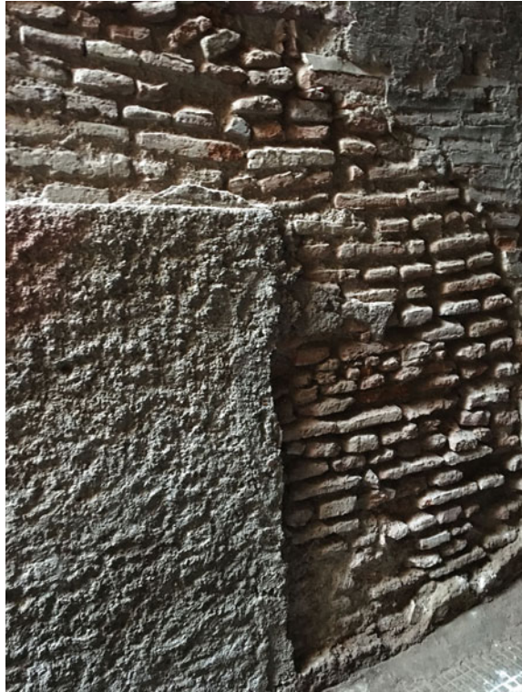
Fig. 4 Brick masonry in Marrakech's medina. Photo: A. Condello, 2019
