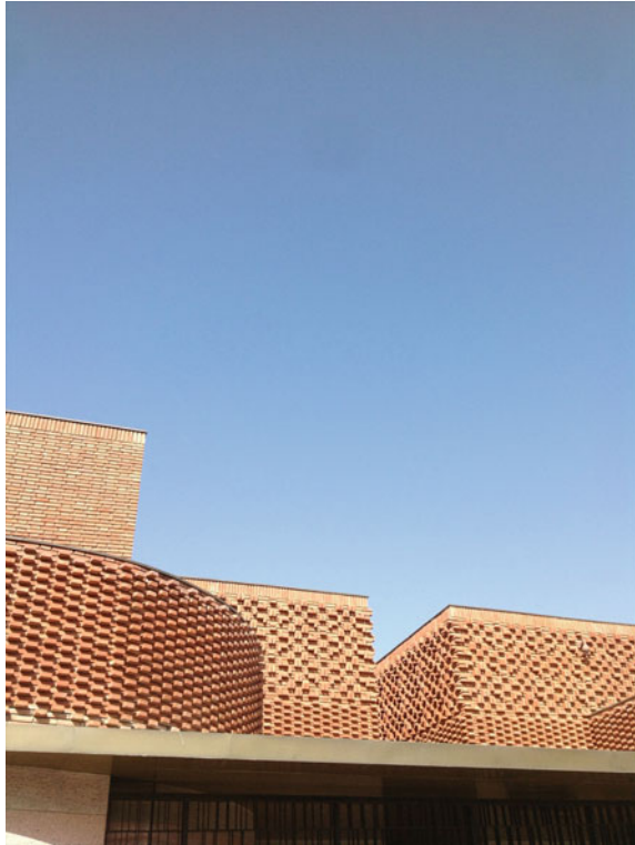
Fig. 8 YSL museum showing three different types of brickwork patterns. Photo: A. Condello, 2019
