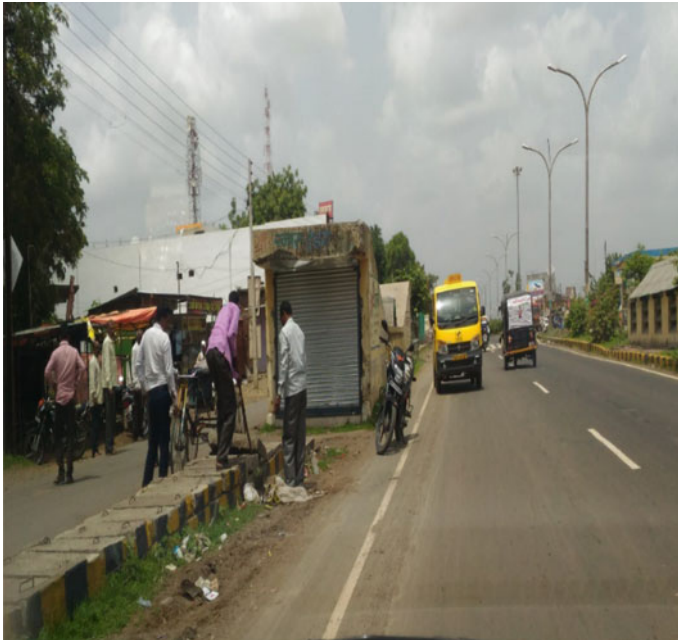
Fig. 7 12.5 km chainage (encroachment)
