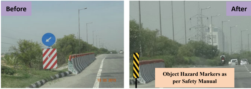
Fig. 6 Traffic signs as per IRC: 67 (2012)
