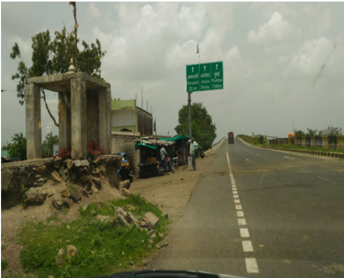
Fig. 9 34 km chainage (dangerous access)
