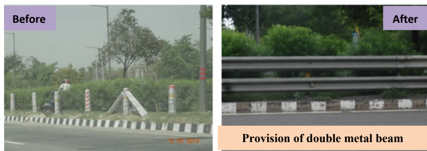
Fig. 3 Before and after the condition of central verge
