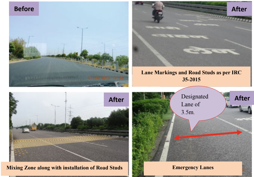
Fig. 5 Road markings and road studs for better night visibility
