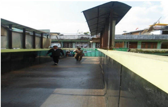
Fig. 2 Location of sidewalk (Site 2)
