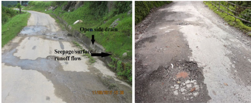
Fig. 4 Road sides allowing water to freely move on the road surface. a Trashingang–Trashiyangtse road (courtesy of Mr. Sonam, Surveyor, Trashiyangtse), b Wangdi–Gelephu Highway (courtesy of Mr. Bishnu Dital, Engineer, Gelephu)
