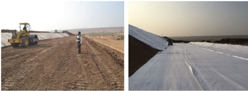
Fig. 6 Rehabilitation works in progress
