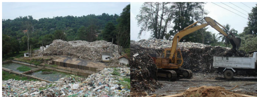
Fig. 20 Small dumps in different locations of the dumpsite
