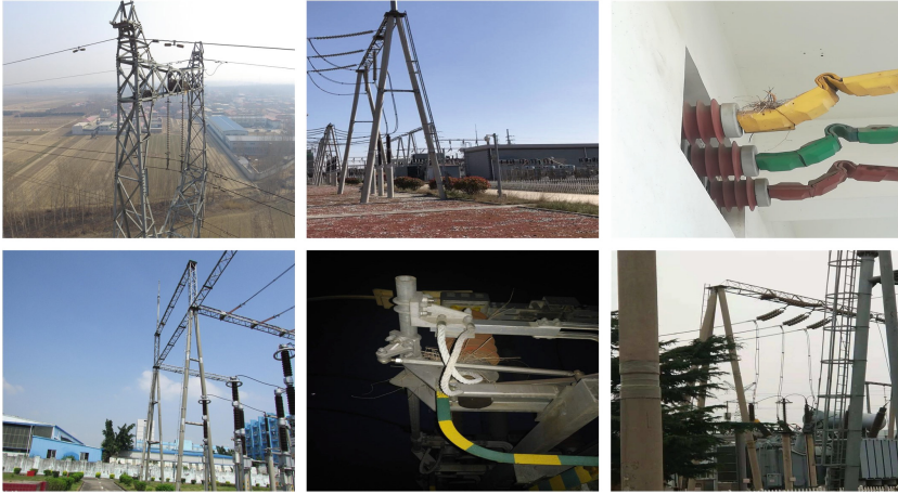
Fig. 1. Bird's nest in the transmission system
