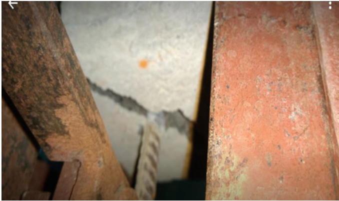
Fig. 15.6 Failure pattern of pull-out test specimen for TMT bars
