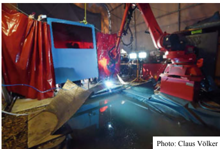
a) Construction site with bridge connection
