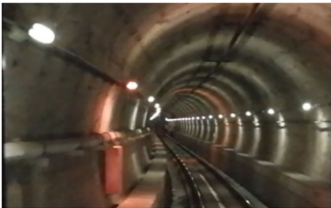
Fig. 1 Surrounding environment of the tunnel line
