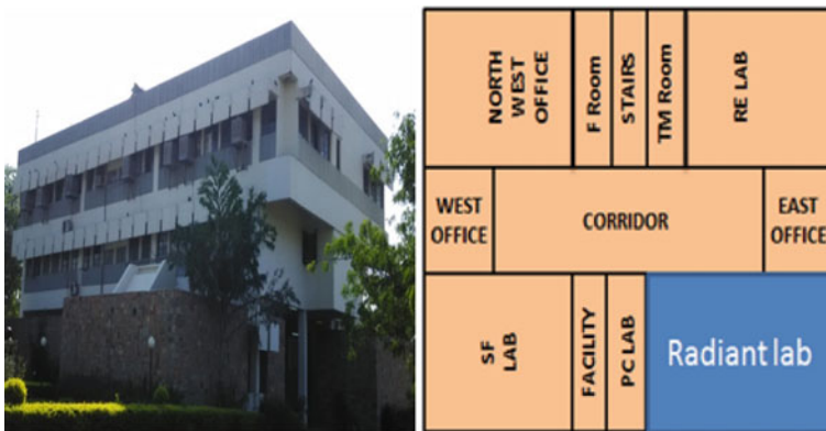
Fig. 7.2 a Old administrative building and b floor plan of second floor
