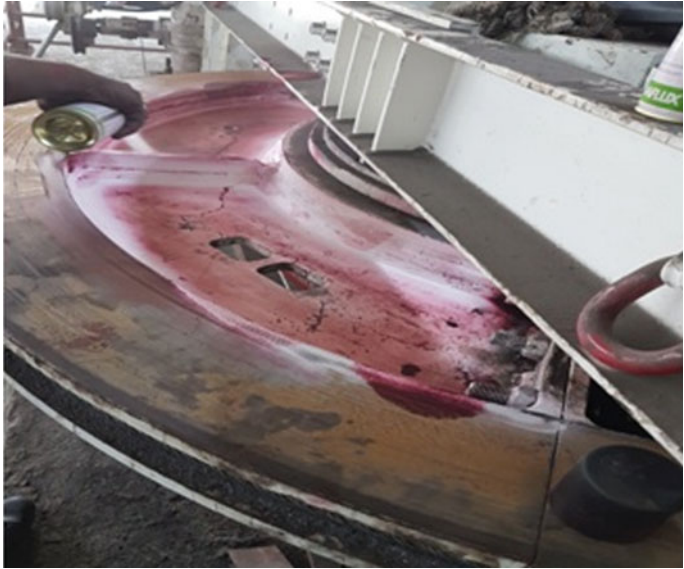
Fig. 3.8 Spraying developer on drive sheave
