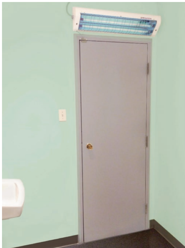
Fig. 75.4 Automatic washroom UV disinfection unit with motion sensors. (Courtesy of Sanuvox Technologies, Montreal, Canada)
