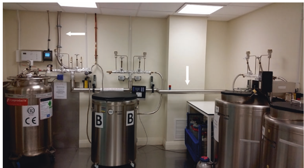
Fig. 65.1 Cryobank pipework. The arrows indicate the pipework required to connect an external LN2 source to multiple vapour phase storage tanks within the cryobank. (Image courtesy of the Knutsford Hewitt Fertility Centre, Liverpool Women’s NHS Foundation Trust, Liverpool, UK)
