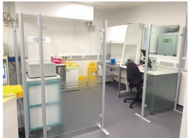
Fig. 74.4 Creating a room within a room using screens. (Courtesy of the Knutsford Hewitt Fertility Center, Liverpool Women’s NHS Foundation Trust, Liverpool, UK)
