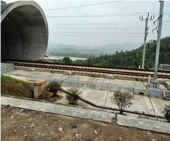
Fig. 1 Test section general situation
