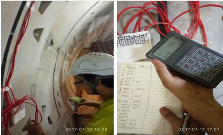
Fig. 5 Shield tunnel grouting pressure measurement site
