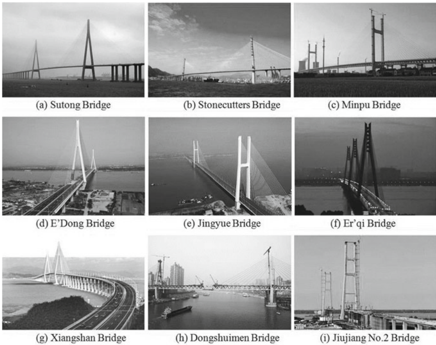
Fig. 2 Recently completed and ongoing large-span cable-stayed bridges in China
