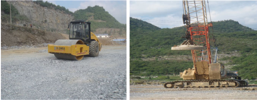
Fig. 2 The rolling-dynamic compaction technology
