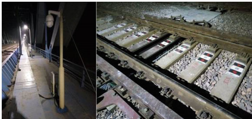
Fig. 8 Sleeper displacement monitoring
