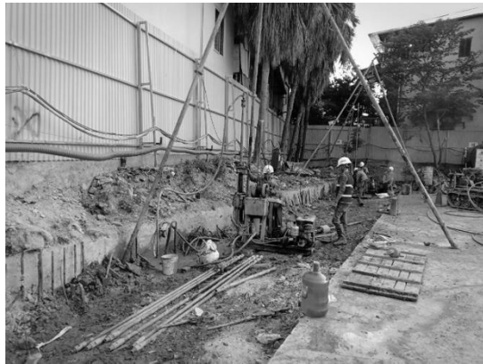
Figure 13. Observation bored hole constructed on site
