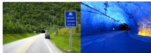
Figure 14. Entrance to Laerdal tunnel (left) and a safety cavern inside World's longest road tunnel (right)
