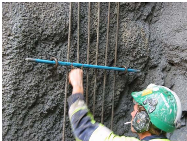
Figure 3. Set-up of RRS comprising of six 16 mm diameter-reinforcing bars.
