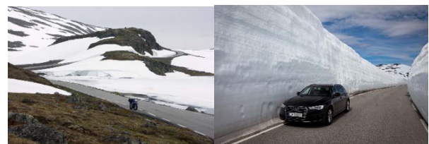
Figure 13. Photos showing the summer road above the Laerdal tunnel (commons.wikimedia.org/wiki)
