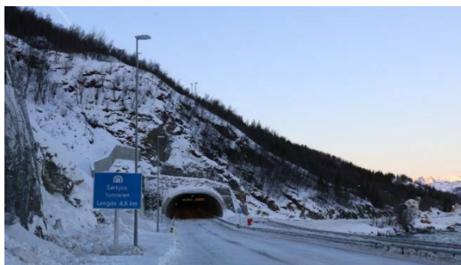
Figure 11. Portal of the South Kjøstunnel
