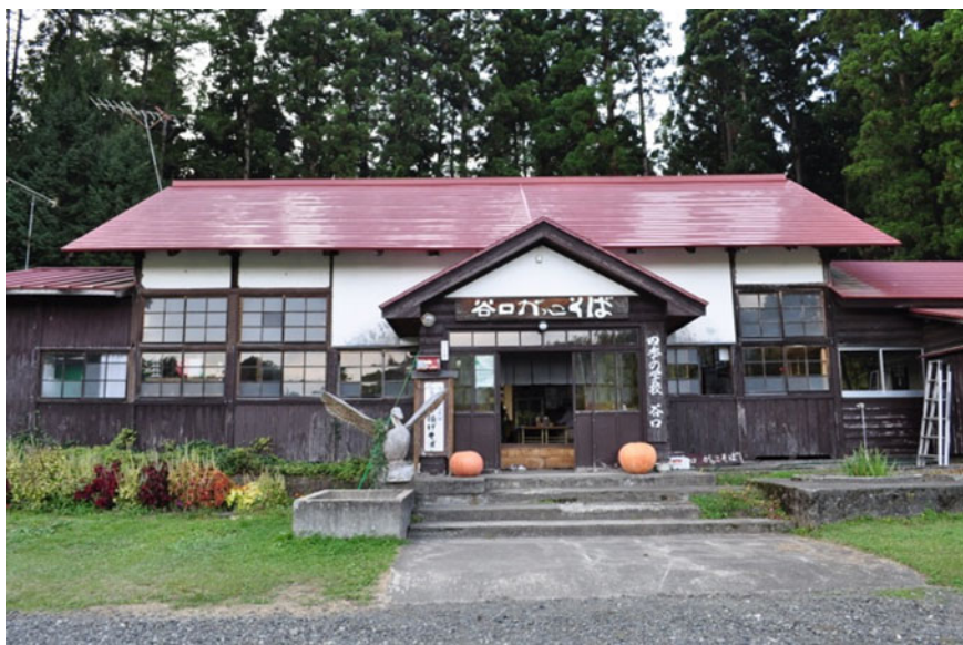
Fig. 2 Exterior of Taniguchi Gakko Soba
