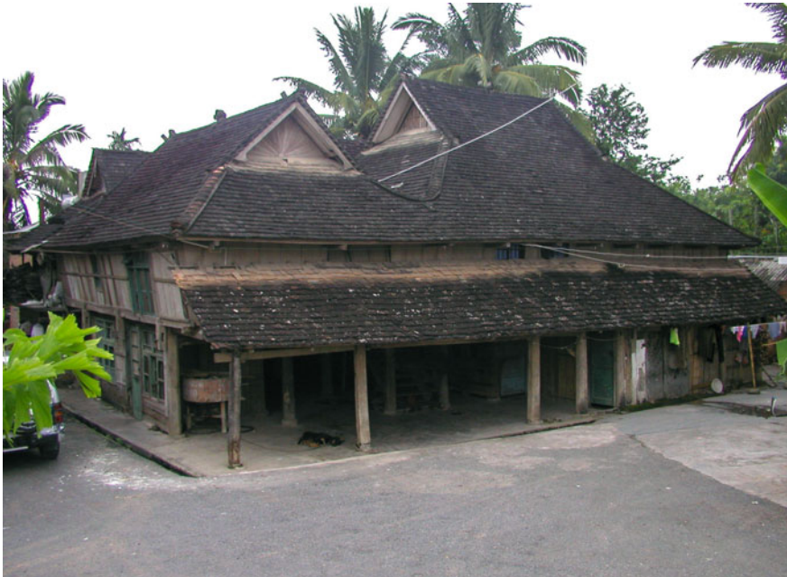
Fig. 3 Traditional raised-floor house of Dai people in Jinghong (2004)
