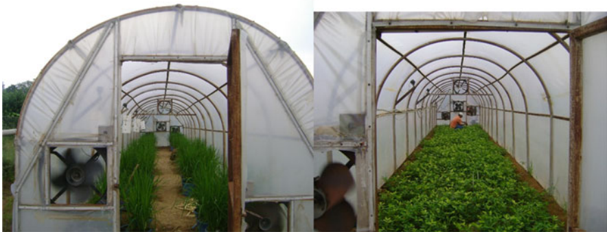
Fig. 3.7 Temperature Gradient Tunnel at ICAR-IARI, New Delhi
