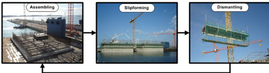
Fig. 2 Floating caisson production cycle
