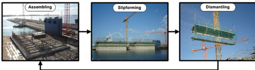
Fig. 2 Floating caisson production cycle
