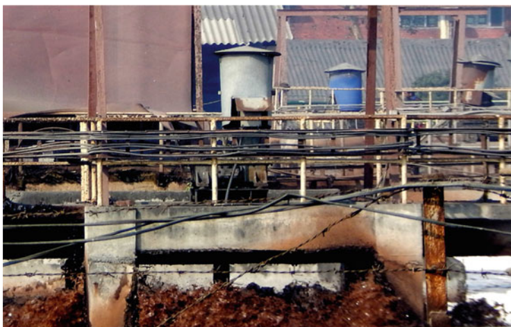
Fig. 1.5 A view of the aerated activated sludge treatment of pulp and paper industry wastewater
