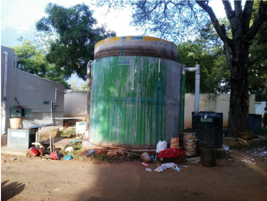
Fig. 3 Full view of existing plant
