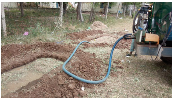
Fig. 3 Composting pit with slurry
