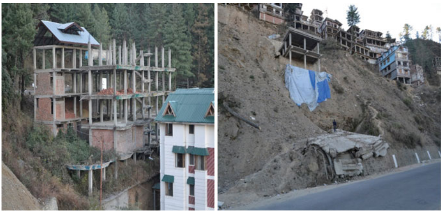
Fig. 2 Construction activity of RC buildings on slopes in Shimla, Himachal Pradesh
