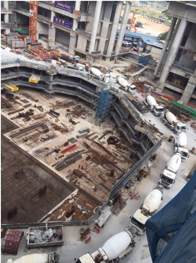
Fig. 2 Typical view on-site during casting with lineup of concrete trucks
