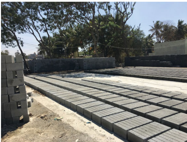
Plate 3 Blocks cast at casting yard
