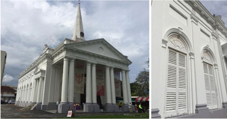
Fig. 1 The building during day time under natural lighting
