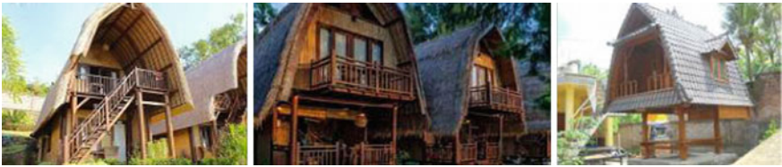
Fig. 10 Modernization of Bale Lumbung house
