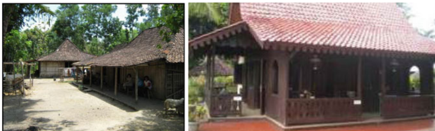
Fig. 4 Original Joglo house (left) and current (right)
