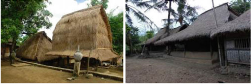
Fig. 9 Traditional Sasak tribal house, Bale Lumbung (left) and Bale Tani (right)
