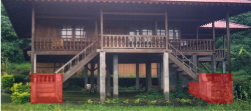
Fig. 7 Use of concrete stairs instead of wooden stairs
