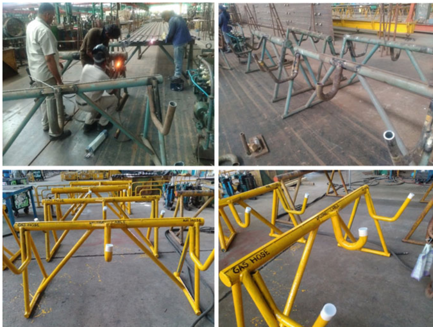
Fig. 6 Fabricating the stand for welding cable, air hose and oxyacetylene gas hose
