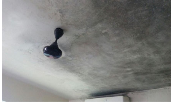
Fig. 30.1 Ceiling of an unconditioned room beneath an air-conditioned zone
