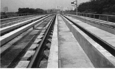
Fig. 1. Plinth structure on the viaducts section
