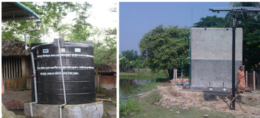
Fig. 9.4 Rainwater harvesting units for safe drinking water ( Source Authors)
