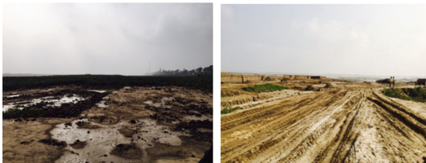
Fig. 8 Initial site conditions
