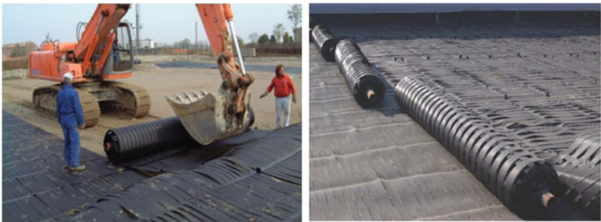
Fig. 12 Installation of transverse and longitudinal geogrids
