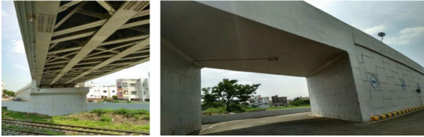
Fig. 4 Existing bridge structure (TC college Baramati to Bhigwan Road, Baramati, Pune)
