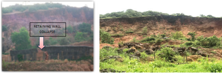
Fig. 2 Ambaji–Fatorda, Goa Landslide site
