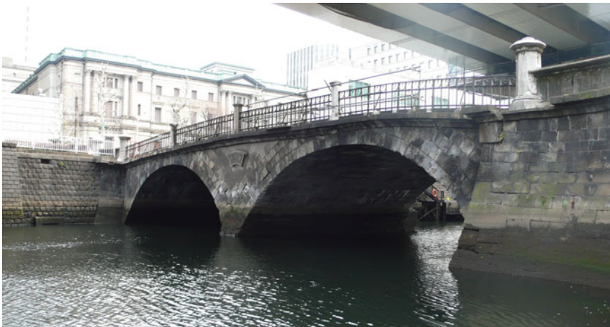
Fig. 1 Tokiwa Bridge (before 2011 Great East Japan earthquake)
