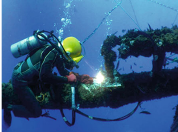
Fig. 14.10 Underwater welding ( http://underwaterweldingschools.org )
