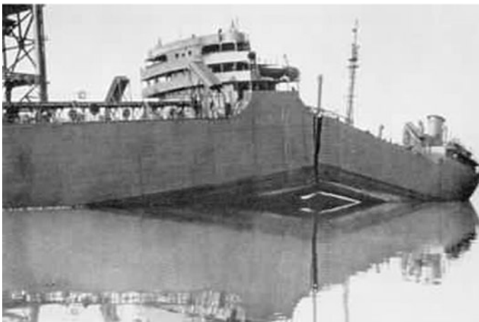
Fig. 13.16 Failure at anchor of the Schenectady tanker ( www.mdp.eng.cam.ac.uk )
