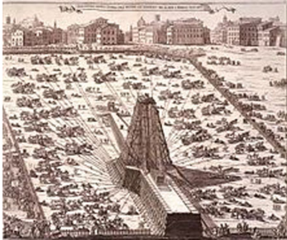
Fig. 3.10 Erection of the Vatican Obelisk in 1586 by means of a lifting tower https://en.wikipedia.org/wiki/List_of_obelisks_in_Rome
