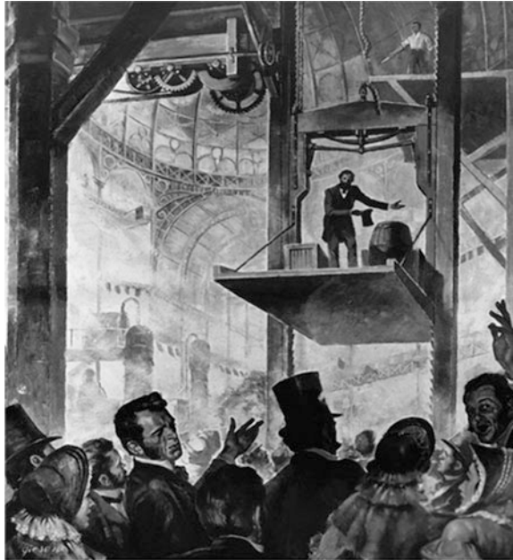
Fig. 4.14 Otis free-fall safety demonstration in 1854 ( 99percentinvisible.org )
