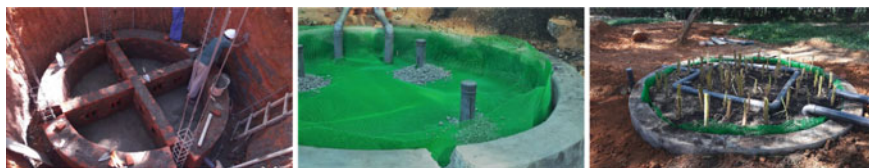
Fig. 2 Construction of the up-scaled ICFiWet system
